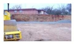
The building contractor at the *ninth grade construction* site has received a favorable plasticity index test on the dirt work. This test measures the amount of moisture in the soil. The next step is to drill multiple
